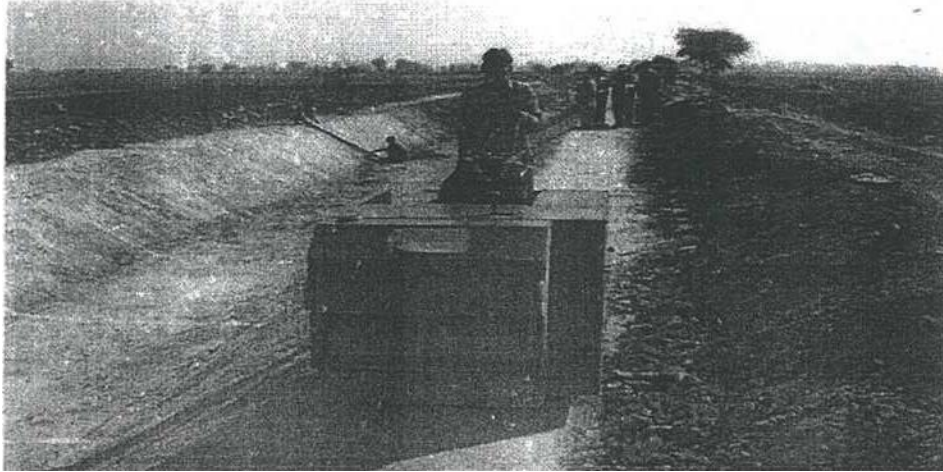
Figure 20 One Metre Wide Vibratory Roller Being Used for Earth fill Compaction
