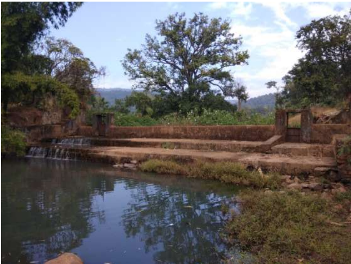
Figure 12 Image of Bisipur MIP Tank during visit
